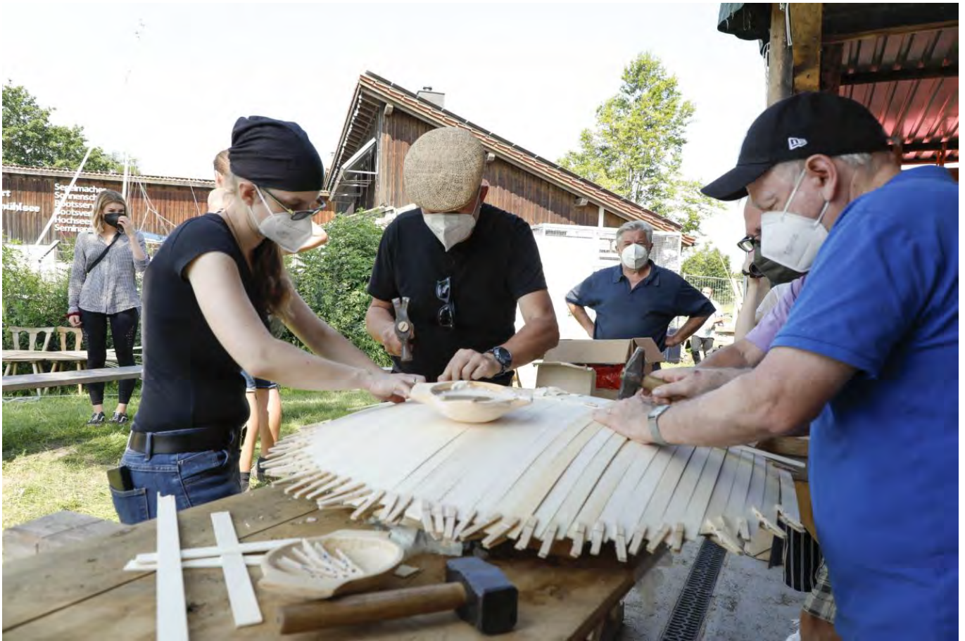
FIG 34. FIRST LAYER OF POPLAR STRIPS ATTACHED WITH CLAMPS, THE SECOND AND THIRD WITH GLUE, TEMPORARILY FIXED WITH LITTLE NAILS UNTIL THE LAYERS ARE DRIED OUT FOR A DAY. PHOTO BY B. DREYER
