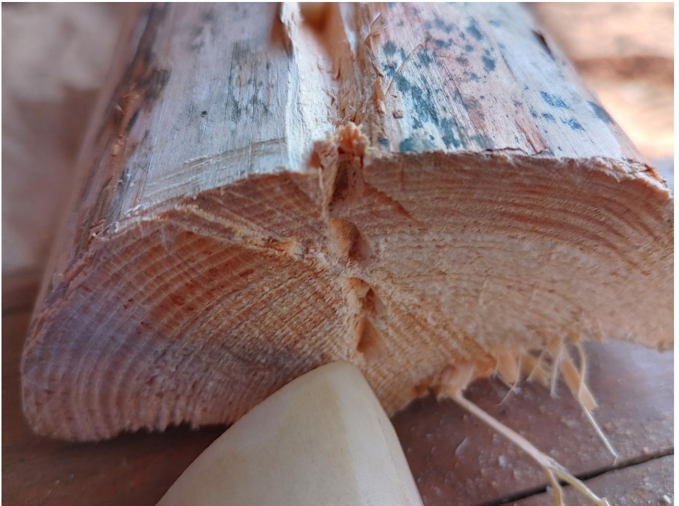
FIG 6A. CREATING A ROW OF INDENTATIONS WITH THE 45 DEGREE BEVELLED TOOL HELPED INITIATE THE SPLIT. A: USING THE TOOL TIP TO MAKE INDENTATIONS. PHOTO BY WOODLAND, 2025
